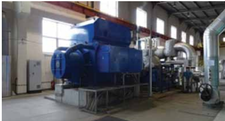
VE-2 16,8 MWe turboagregatas
